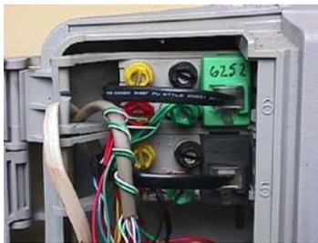
Bring one of your phones outside, or obtain buttset at a hardware store, home store, electrical supply or electronics store. Unplug the short-wired phone plug from the jack in the interface corresponding to your phone line and plug in the phone (or buttset). A dial tone (or proper lighting sequence) will tell you that the phone company is not at fault. If you receive no dial tone, get on the cell phone and call the repair service!
